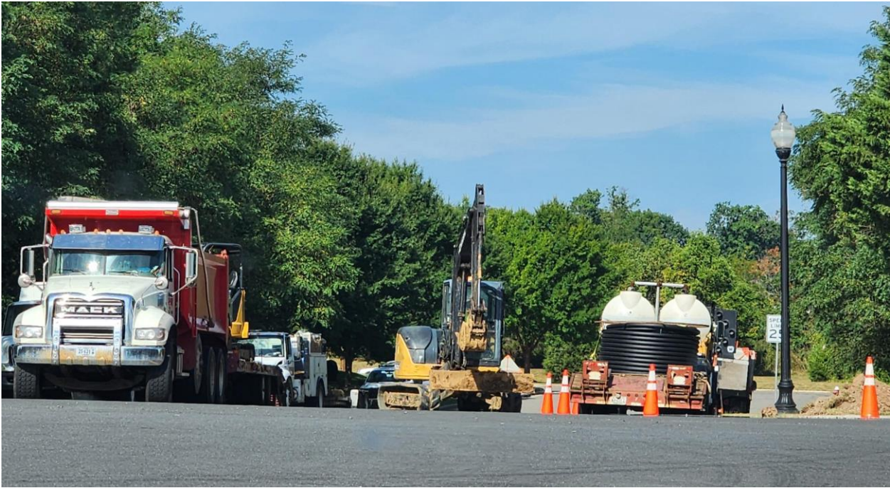
8/30/23: Photo - showing infrastructure installations underway.
