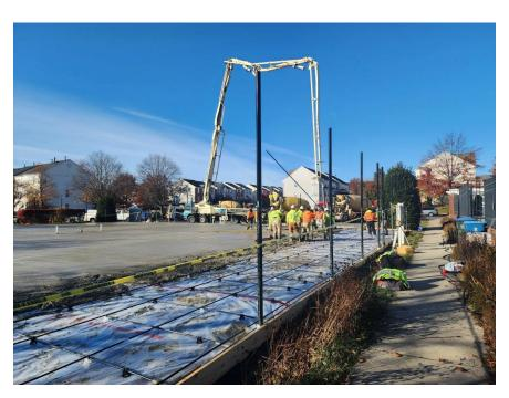
**11/8/2023:** The photo below shows the moisture barrier and tension rods in place at the **Town Hall** courts. The concrete pour is scheduled for 11/14, weather permitting.
