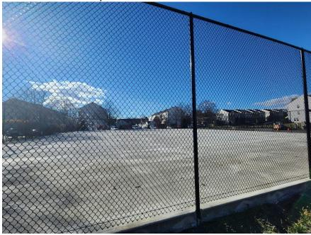
**11/14/2023:** The concrete was poured today at the **Town Hall** courts. Plastic and concrete blankets will be laid over the surface. Soon we'll see the fencing go up and upon delivery the lighting will be installed.
