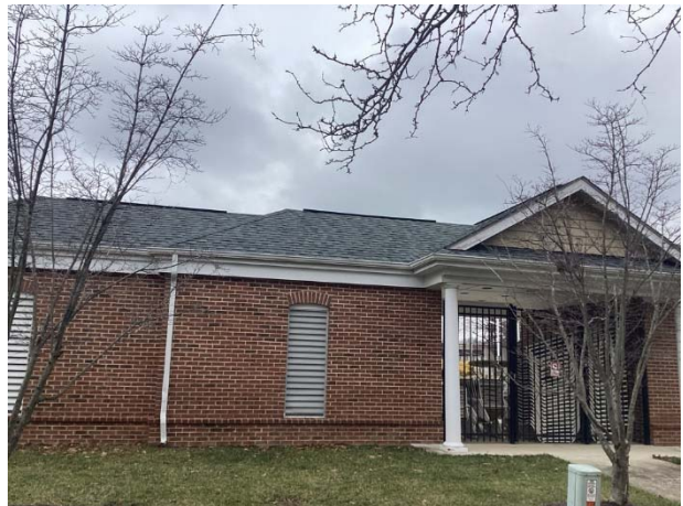
Roof overview at splash pool
