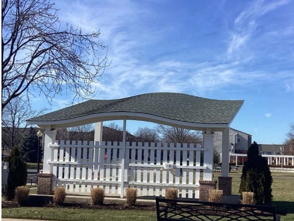
Town Hall bandstand roof
