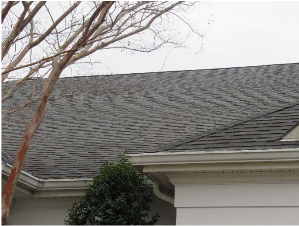
Asphalt shingle roof overview
