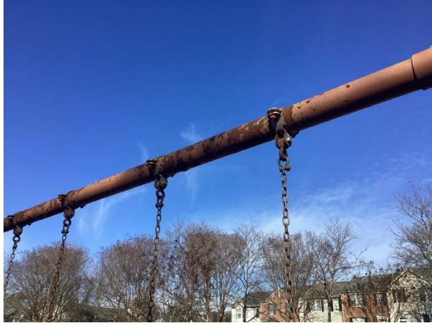
Equipment finish deterioration and rust
