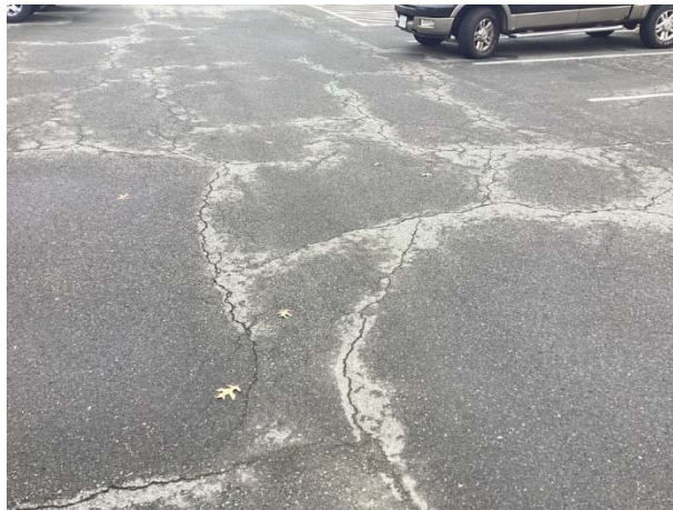
Pavement cracks
