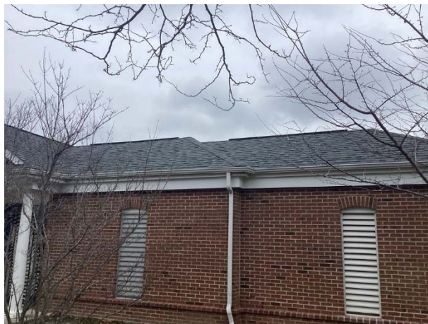
Roof overview at splash pool
