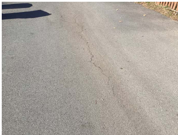
Pavement cracks
