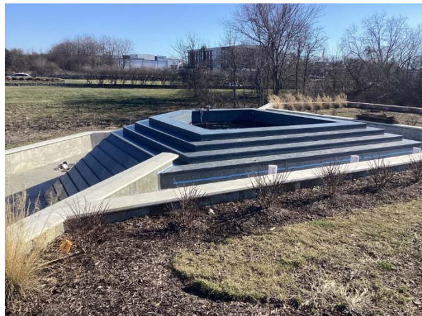
Entrance monument fountain at front entrance
