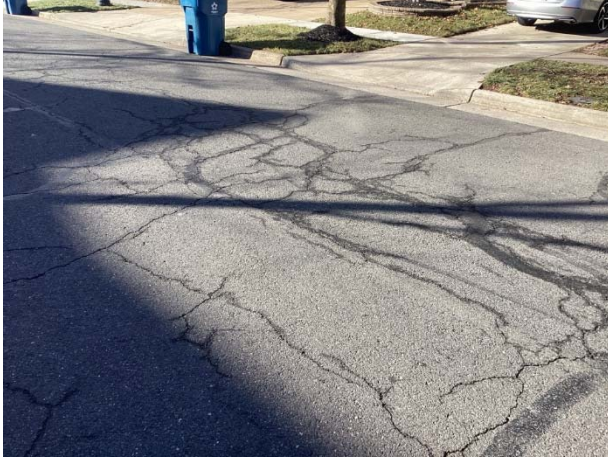
Pavement cracks
