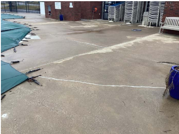
Concrete pool deck overview
