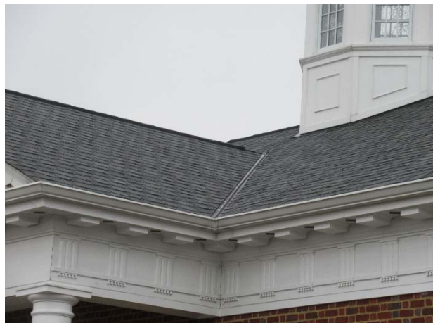
Asphalt shingle roof overview
