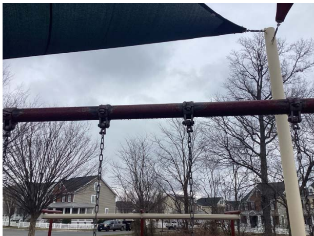
Equipment finish deterioration
