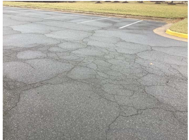
Pavement cracks
