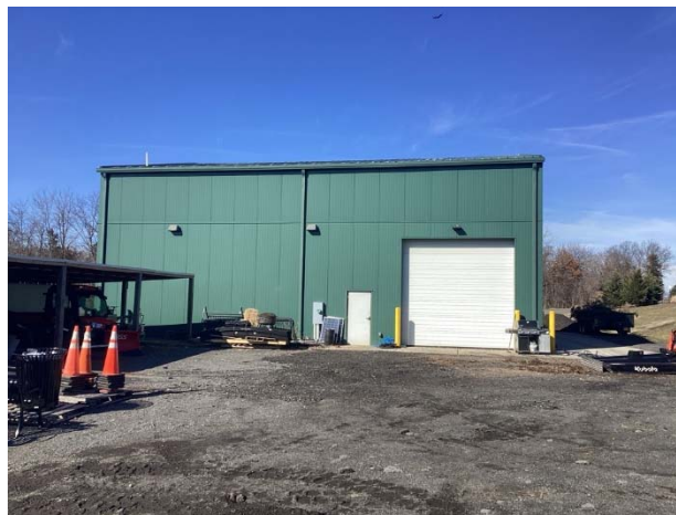
Maintenance building overview
