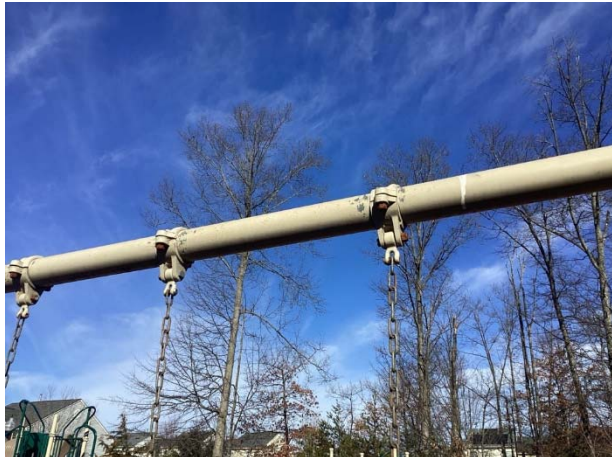
Fastener rust and finish deterioration
