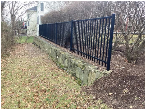
Retaining wall and fence
