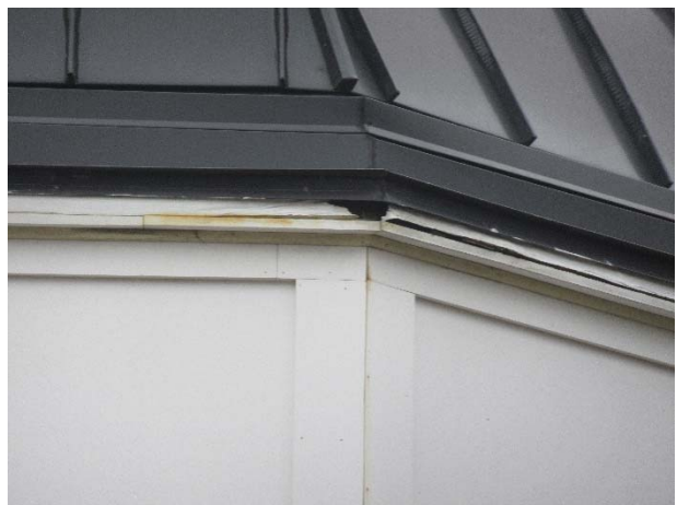
Trim deterioration
