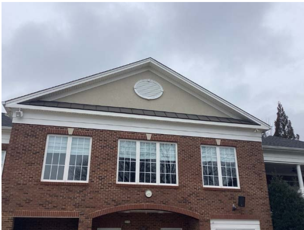
Metal roof overview
