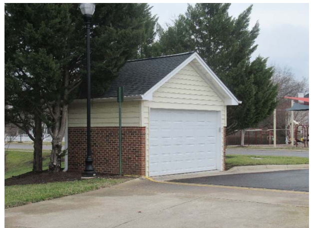
Shed overview – Note: roof replacement included with main building roof replacement
