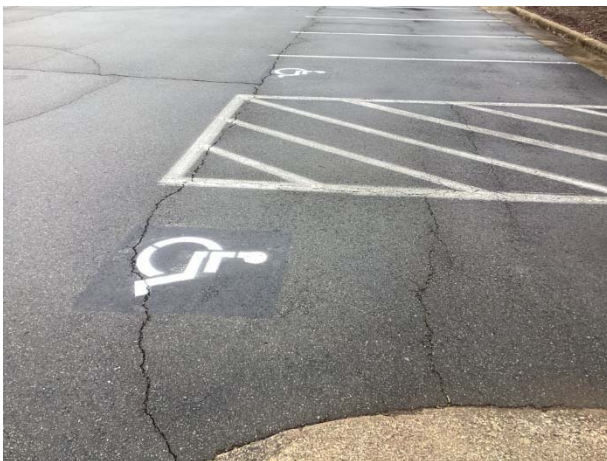
Pavement cracks
