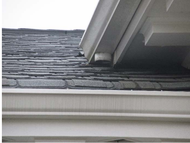
Downspout discharge directly onto lower elevation roof
