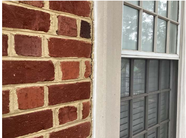
Mortar cracks
