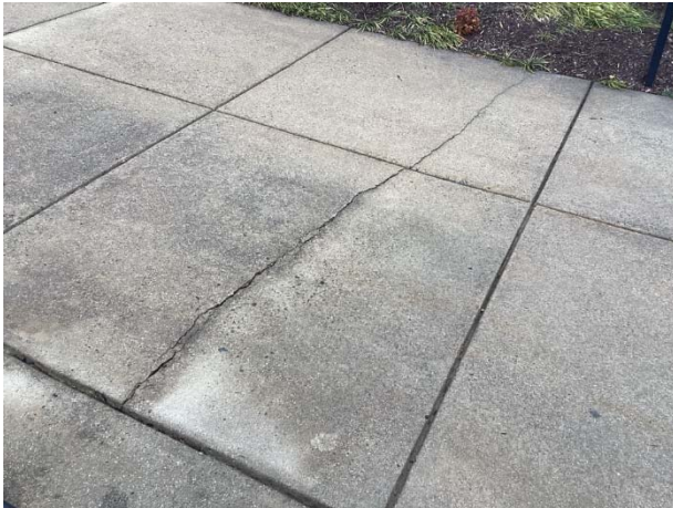
Sidewalk cracks
