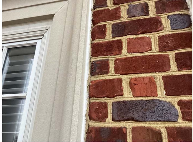
Mortar cracks
