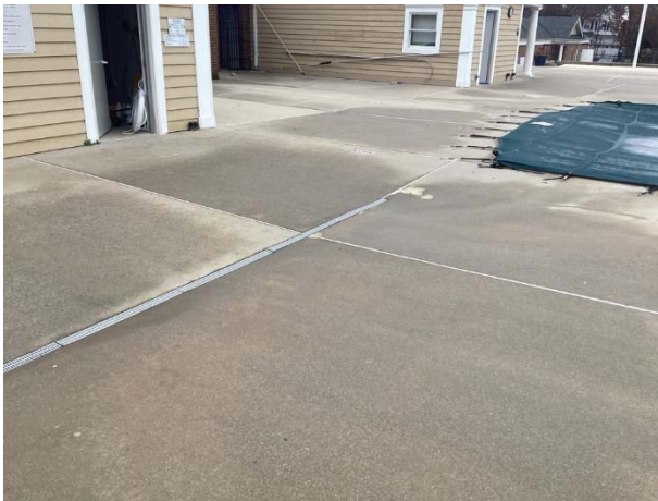
Concrete pool deck overview
