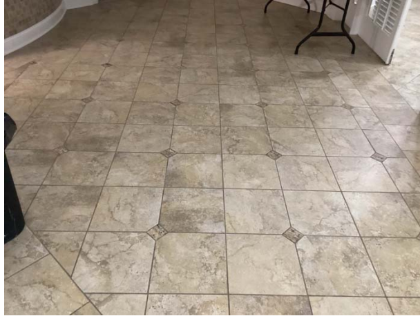
Tile floor coverings
