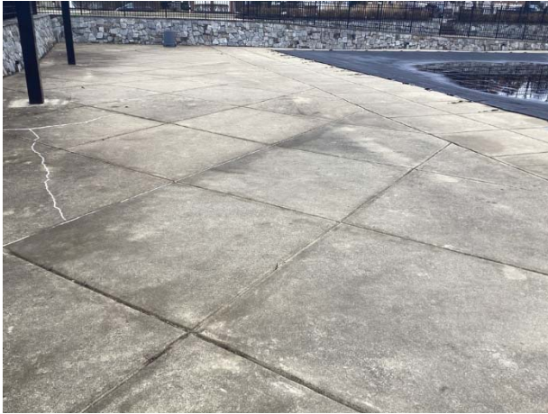
Concrete pool deck overview
