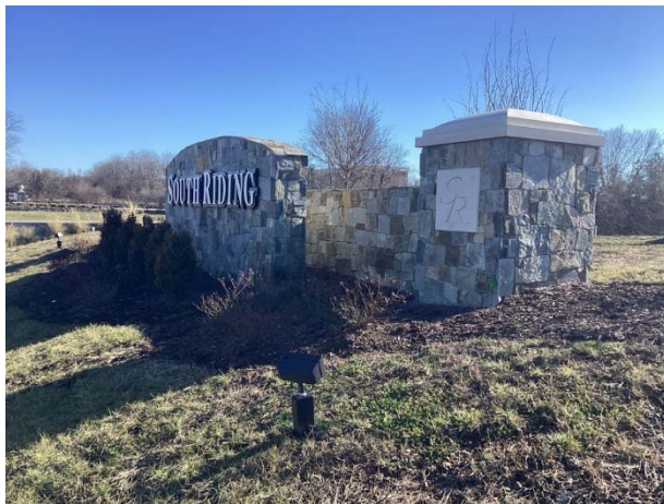
Entrance monument at front entrance
