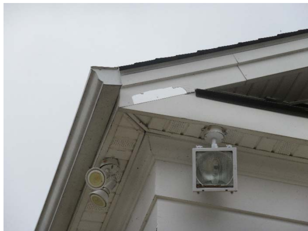
Trim deterioration
