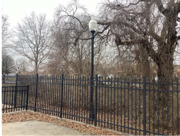
Light pole and fixture
