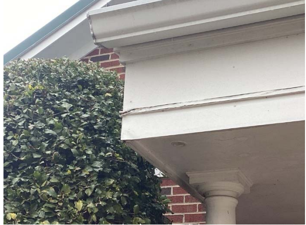
Trim deterioration
