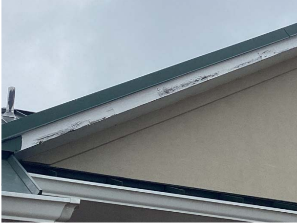
Trim deterioration
