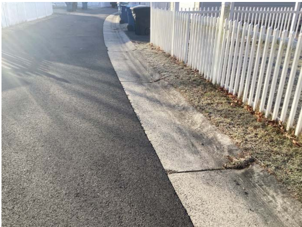
Concrete curb and gutter
