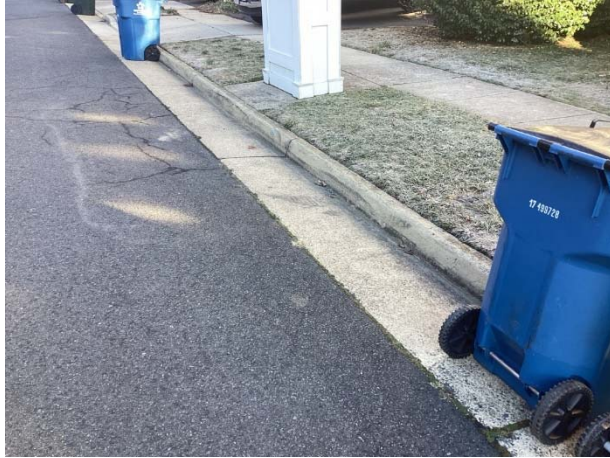
Concrete curb and gutter
