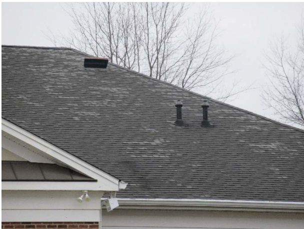
Asphalt shingle roof overview
