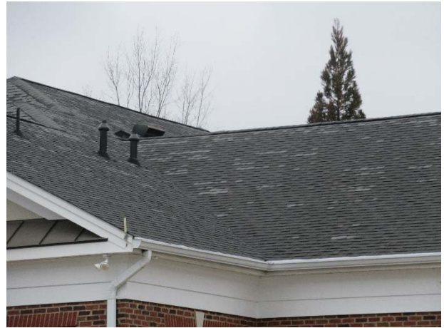
Asphalt shingle roof overview
