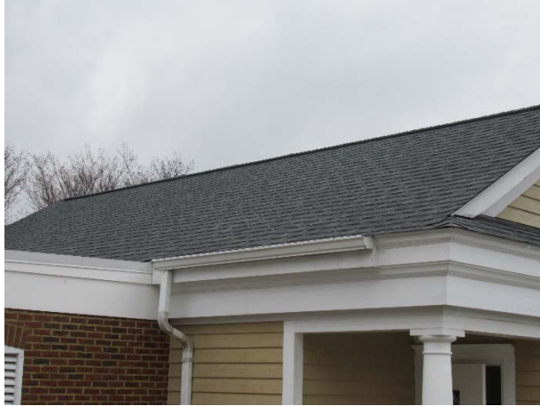
Roof overview at main pool
