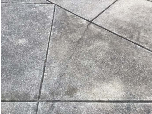
Concrete cracks
