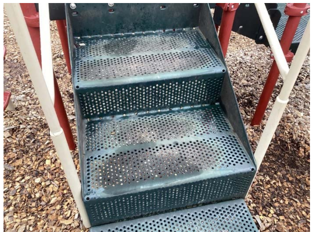
Equipment finish deterioration
