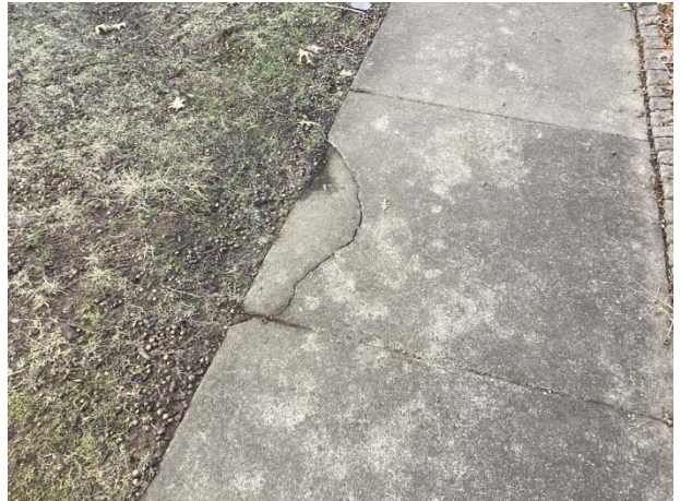
Sidewalk cracks
