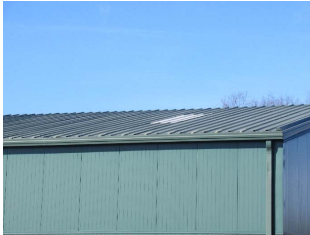
Metal roof overview
