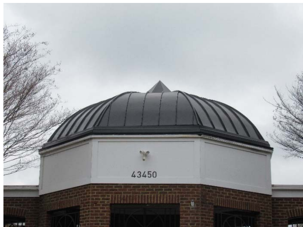
Metal roof overview
