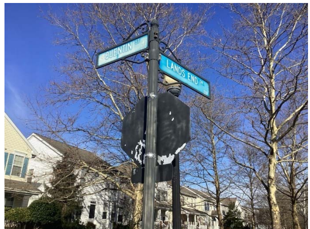
Sign finish deterioration
