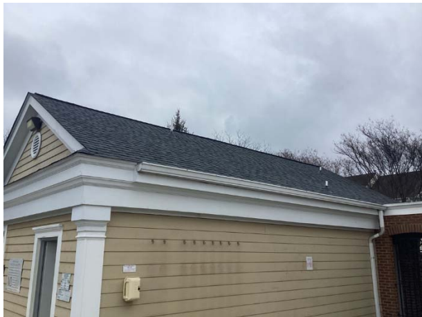
Roof overview at main pool
