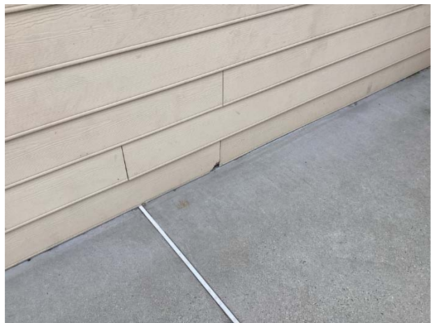
Siding damage
