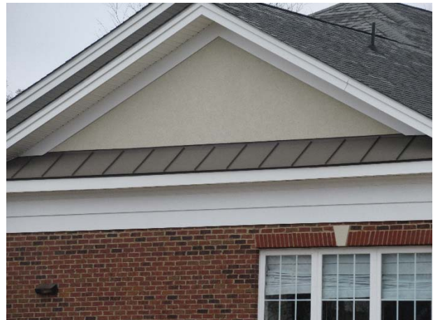
Metal roof overview
