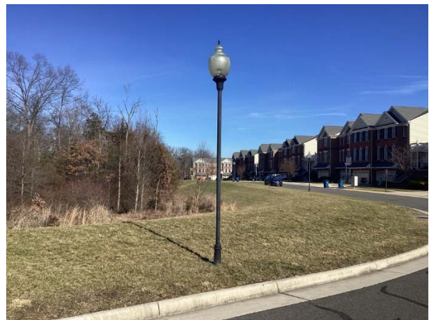
Light pole and fixture
