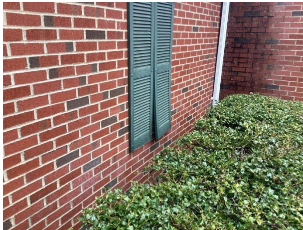
Shutter displacement
