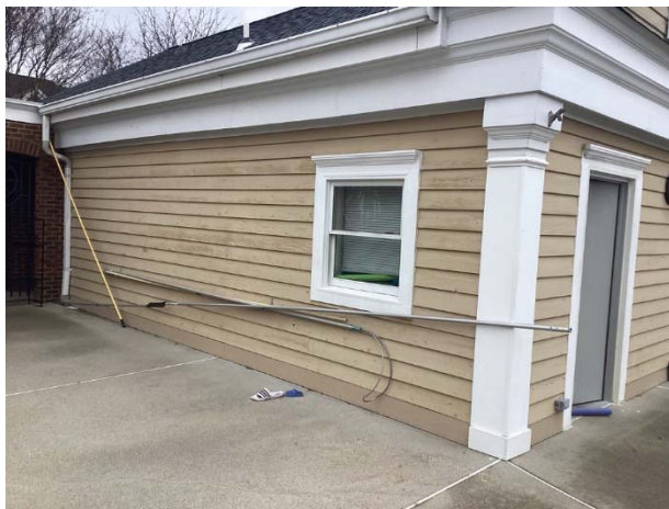
Siding and trim overview
