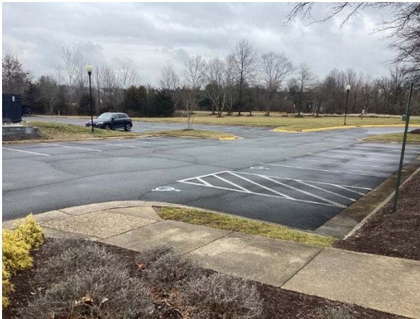
Pavement overview at Meadows pool house
