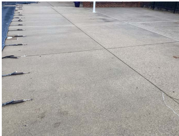
Concrete pool deck overview
