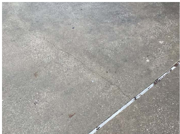
Concrete cracks
