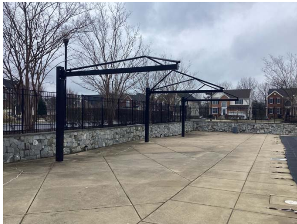
Shade structure overview
