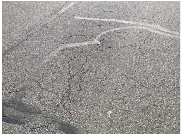
Pavement cracks
