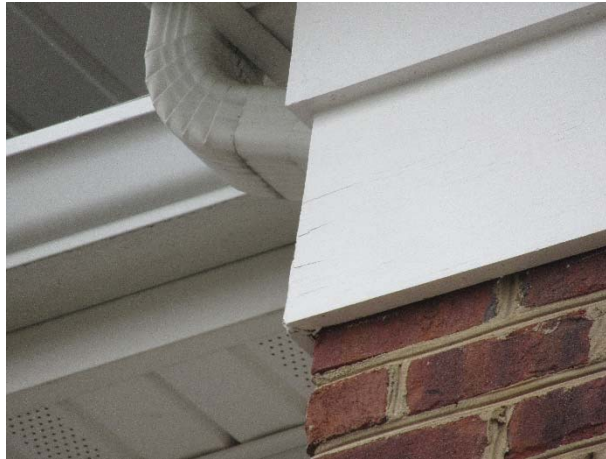
Trim deterioration
