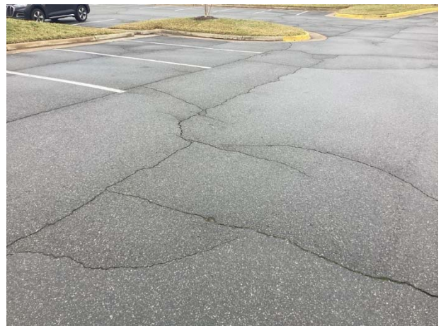
Pavement cracks
