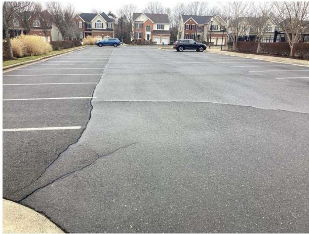
Pavement overview at South Riding Center
