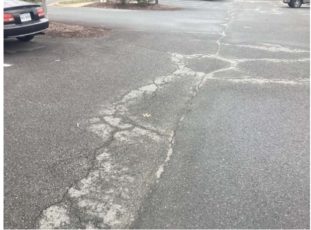
Pavement cracks
