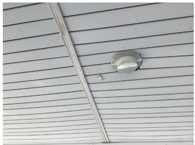
Soffit damage
