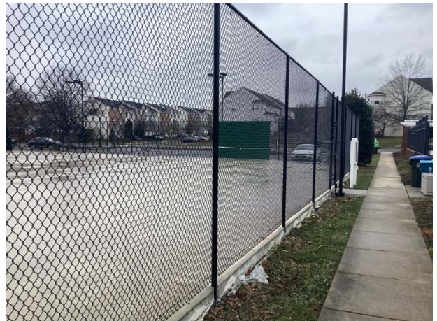
Chain link fence at Town Hall
