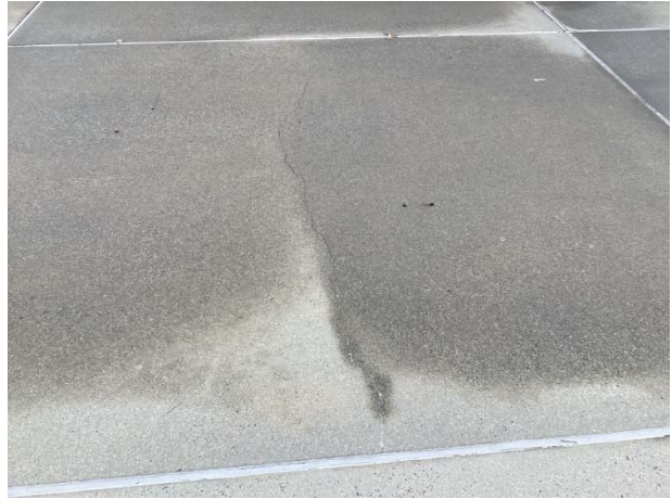
Concrete cracks
