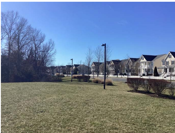
Light poles and fixtures
