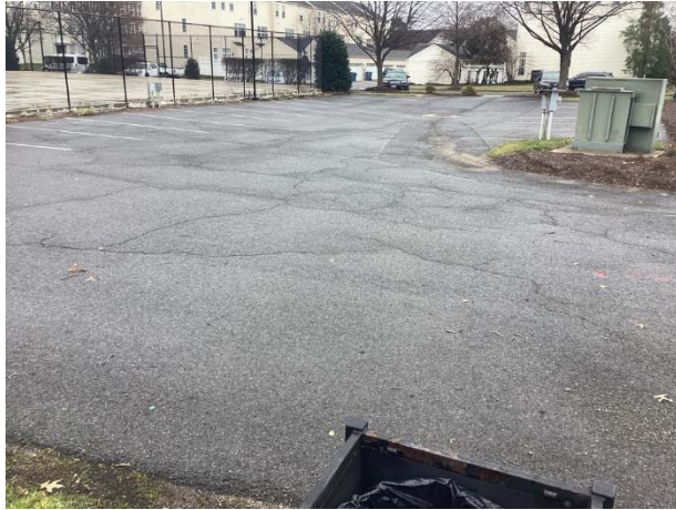
Pavement overview at Town Hall
