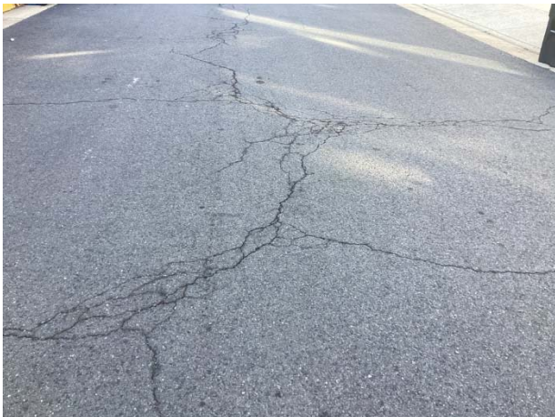
Pavement cracks
