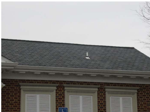
Asphalt shingle roof overview
