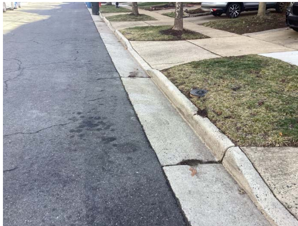
Concrete curb and gutter
