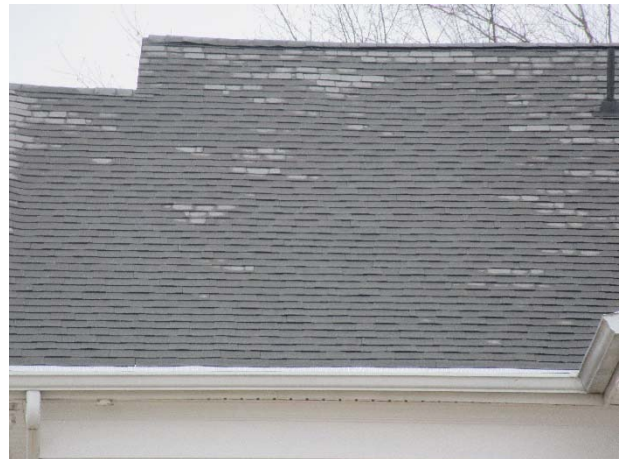
Asphalt shingle roof overview
