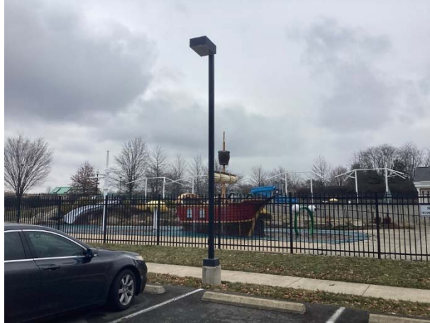
Light pole and fixture
