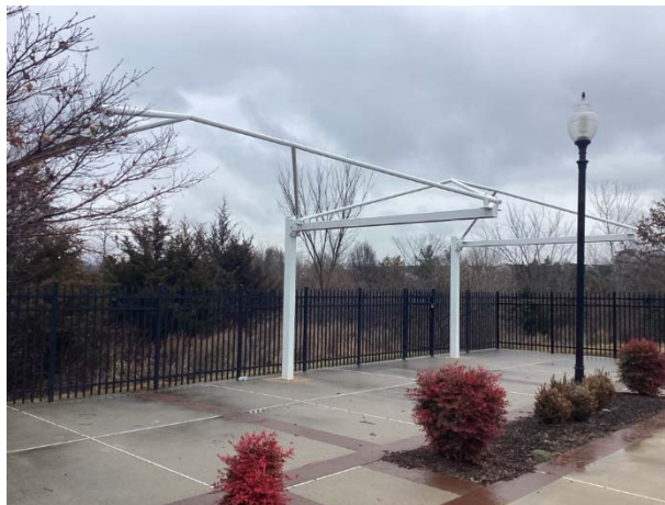
Shade structure overview
