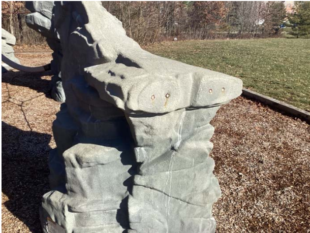
Fastener rust and equipment finish deterioration
