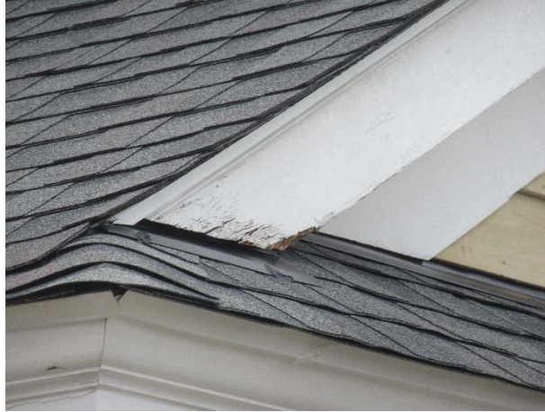
Trim deterioration
