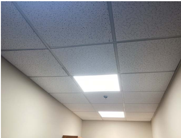
Acoustical ceiling tiles
