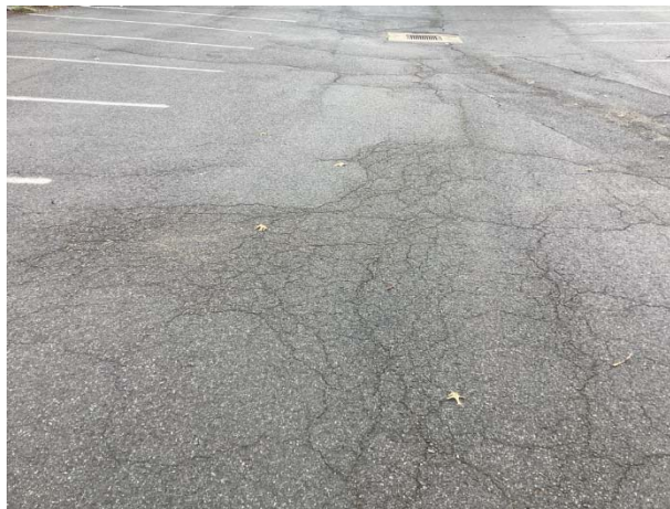
Pavement cracks
