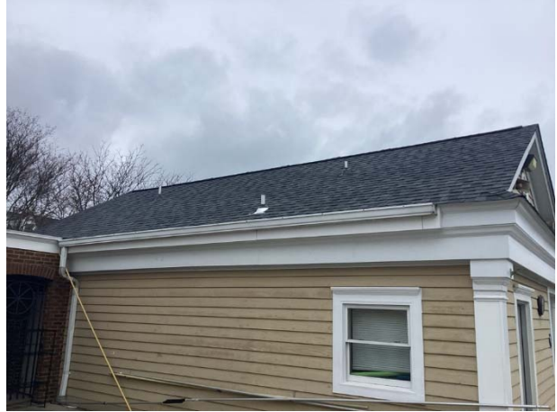
Roof overview at main pool
