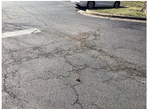
Pavement cracks
